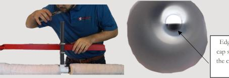
Edge of white cap should be in the center of the t-riser
