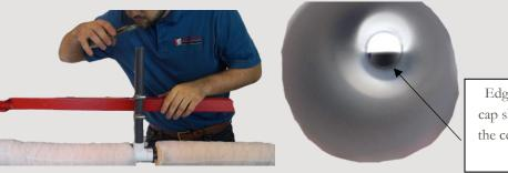
Edge of white cap should be in the center of the t-riser
