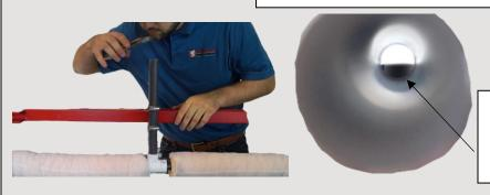
Edge of white cap should be in the center of the t-riser
